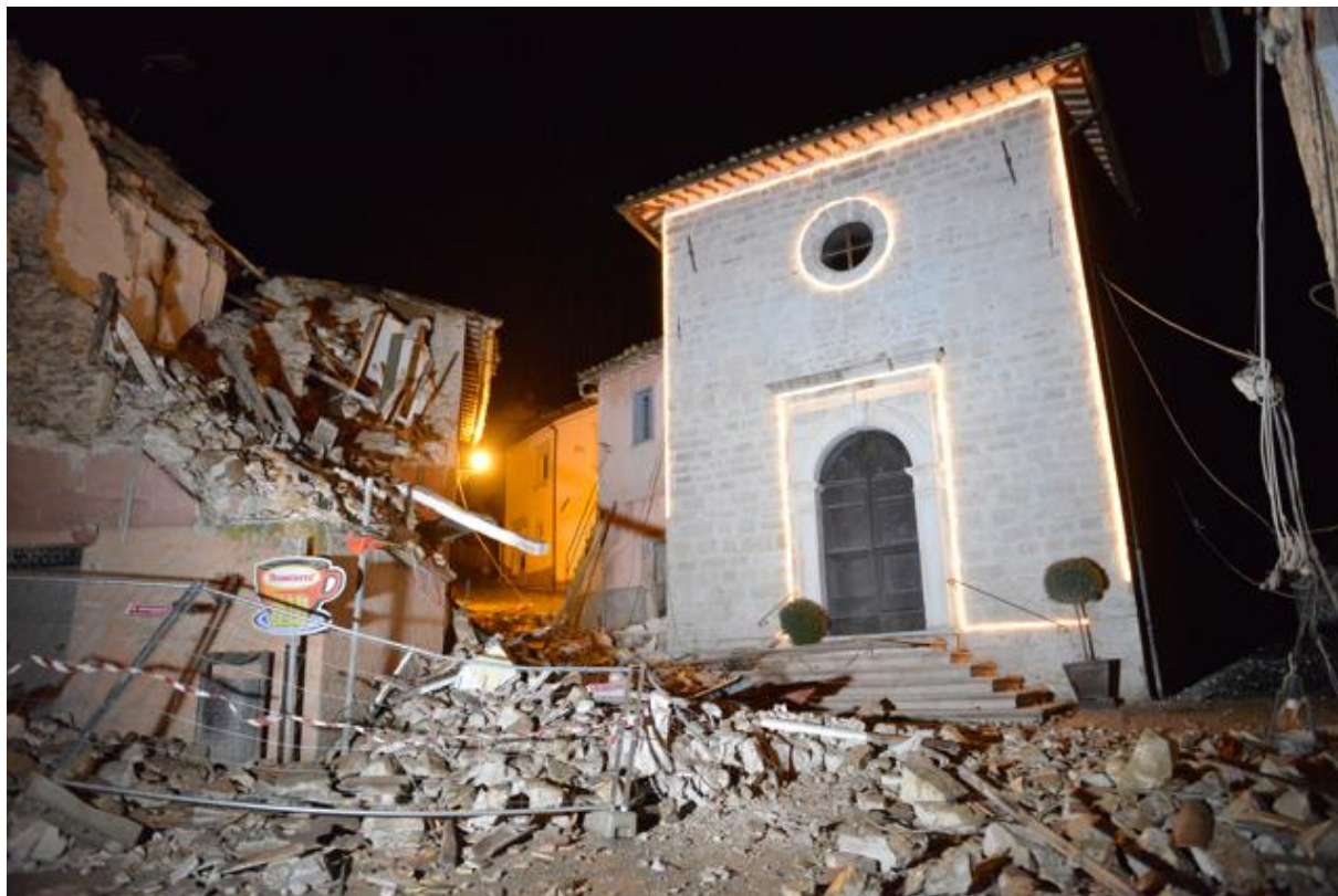
Figure 34: An area of the center after the earthquake in 2016 [118]
